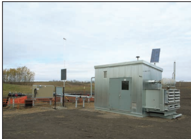
■ The package has been engineered for placement on an engineered gravel pad in remote locations. To further reduce atmospheric emissions, solar panels incorporated into the unit use the sun's energy for operating the control and gas detection systems.
